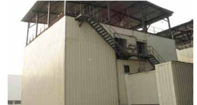
Bag filter for boiler of Suqian Bio-mass Generation Project
