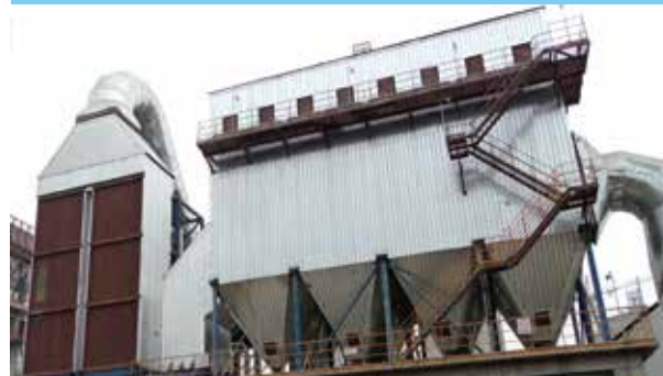
Bag filter and air air heat exchanger for cooler of Sinoma Hanjiang Cement Plant( 2500t/d)
