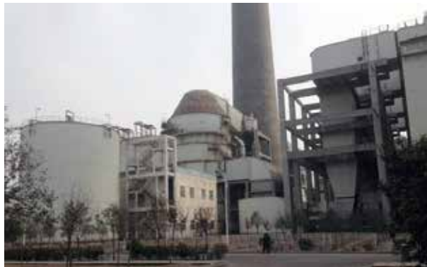
2×600MW uint flue gas desulfuriztion project
