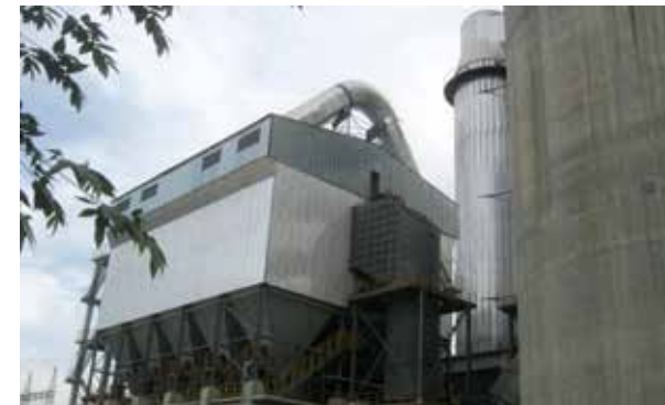
Bag filter for kiln of Malaysia Bahau Cement Plant (5000 t/d)
