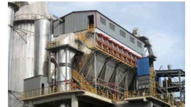
Bag filter for coal mill of Malaysia Bahau Cement Plant (5000 t/d)
