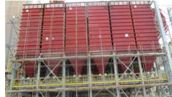
Module Bag Filter for Kiln of Caapora Cement Plant of Lafarge Brazil (4000 t/d)
