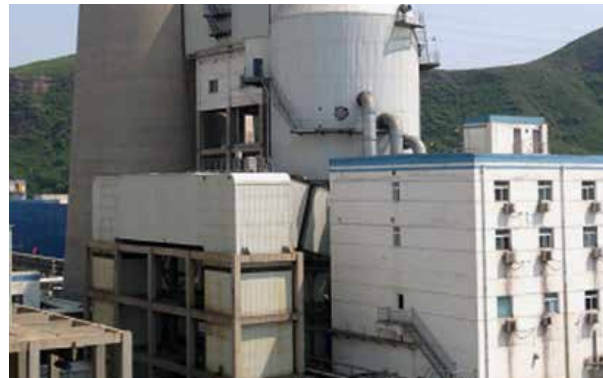
300MW uint flue gas desulfuriztion project
