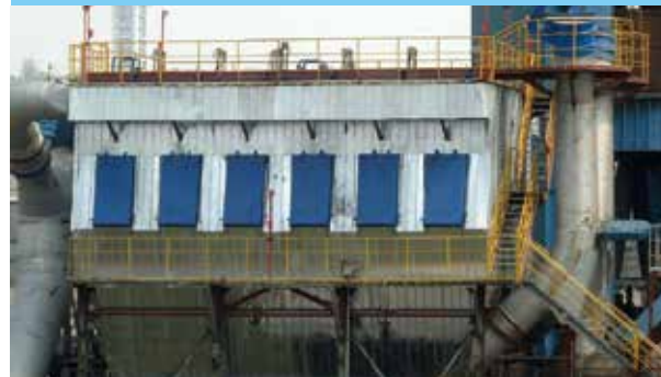
Modification of coal mill bag filter (28t/h) for DOCC-Improving traditional coal mill bag filter with TDM pulse jet technology
