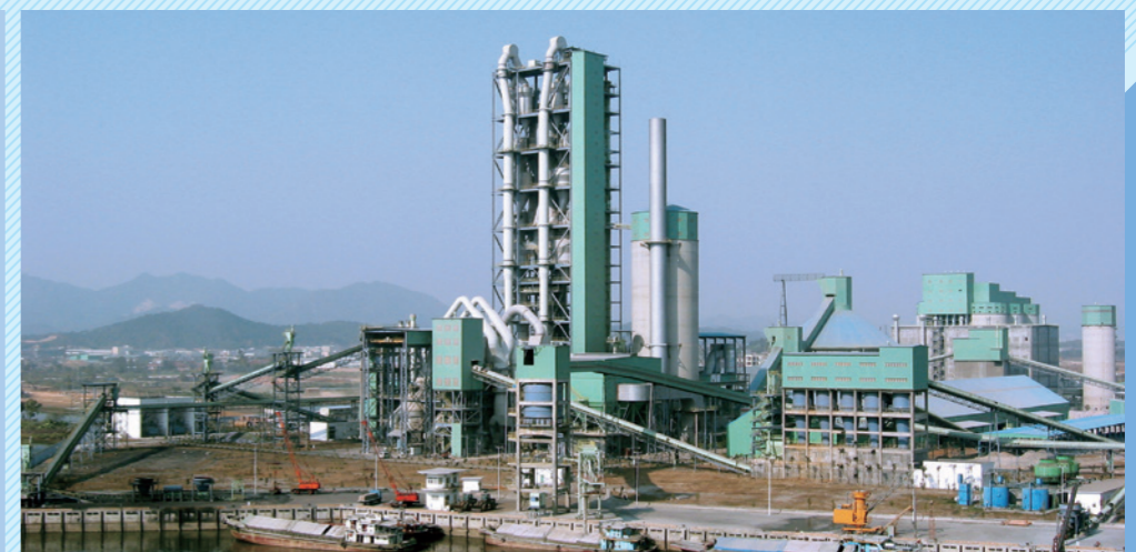
Heidelberg Guangzhou Sludge Treatment Project, dry sludge feeding into cement kiln for incineration, replacing partial raw materials and fuel, also achieving the complete sludge harmless disposal, which is the international advanced level, operated in 2008
