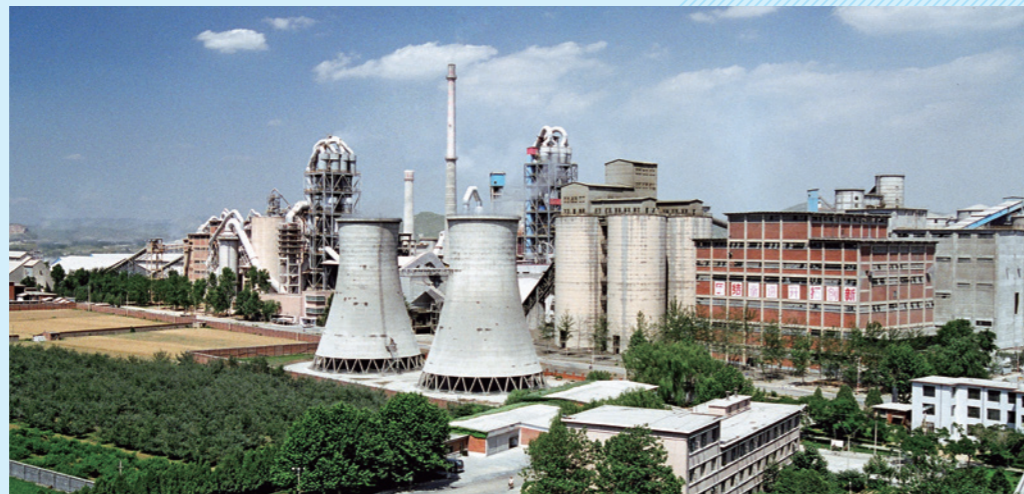
Hebei Jidong Cement Plant Line 2, China's first localized equipment 4,000t/d production line, operated in 1996
