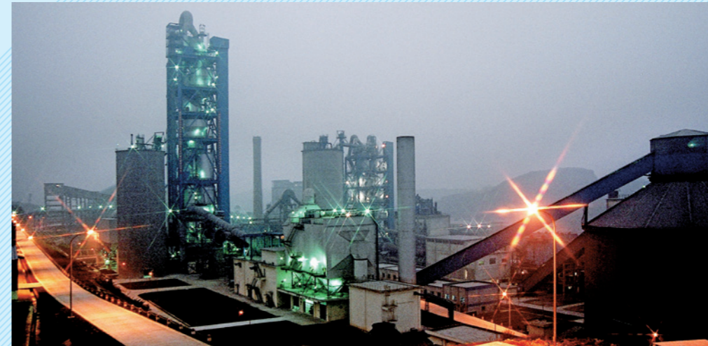
Tibet Gaozheng Building material Co., Ltd. 2,000t/d Project, the highest altitude new dry process cement production line in the world (elevation is 3720 meters) , operated in 2004
