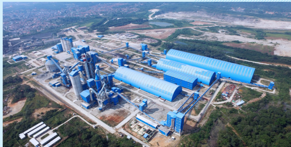
Indonesia BATURAJA 5,000t/d cement production line EPC project, complete all workshop performance tests 137 days in advance of contract and obtain PTCC(PAC) certificate issued by owner, the fastest construction period in Indonesia's history, operated in January 2018.
