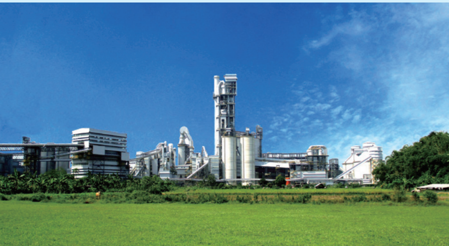
Heidelberg INDOCEMENT- P14 10,000t/d Project, our company's first EU standard overseas ten-thousand-ton-level EPC project, operated in 2016
