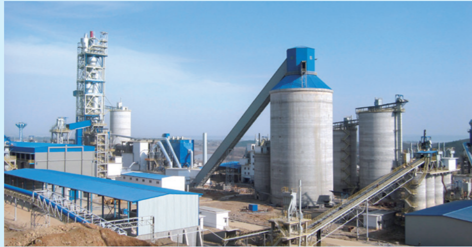
Anqing Aalborg 1,300t/d White Cement Plant, the largest scale white cement production line in the world, operated in 2009
