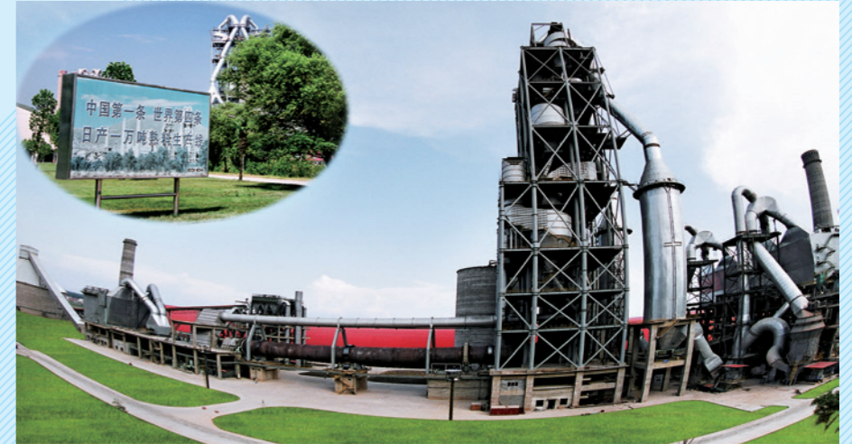
Conch Zongyang Cement Co., Ltd Phase 3 Line 1, China's first 10,000 t/d new dry process cement production line, operated in 2004
