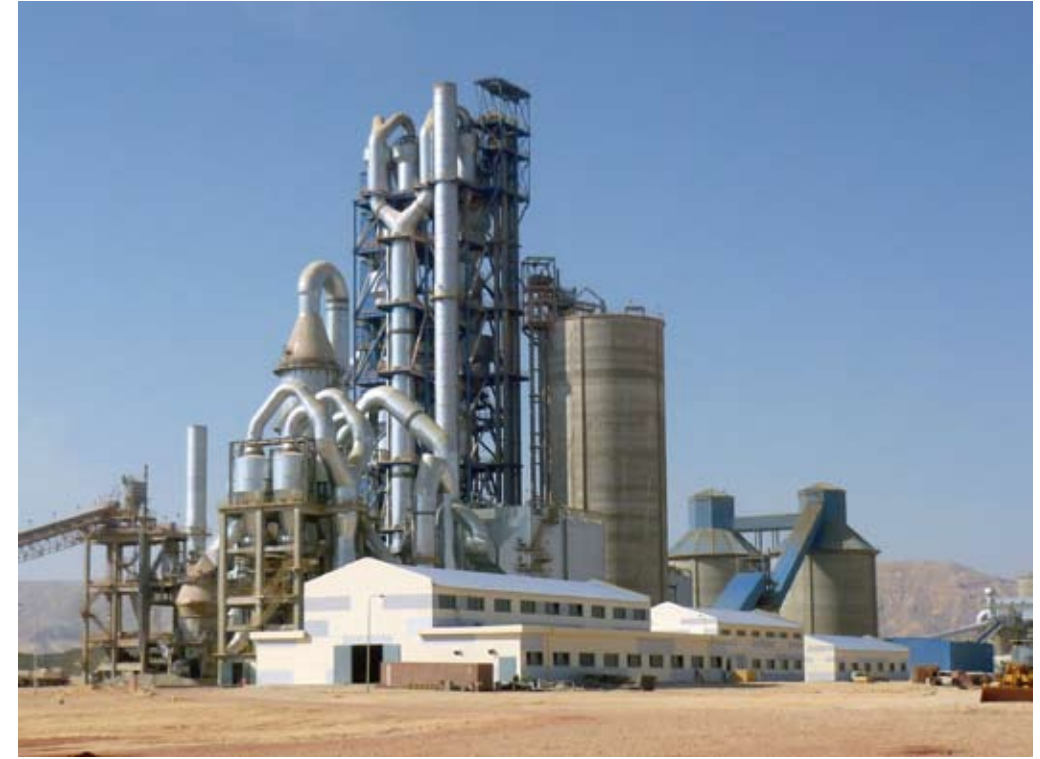
未来新型干法硫铝酸盐水泥生产线 Future Sulphoaluminate Cement Production Line
