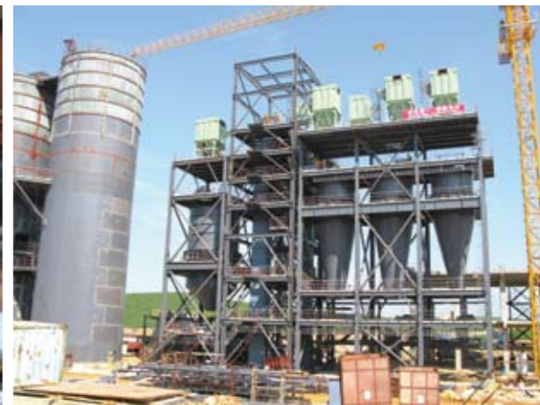
▲ 吊装作业 Lifting operations
