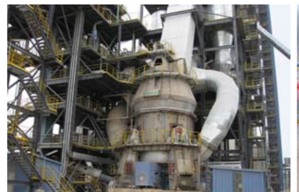
▲ 原料磨安装 Raw material grinding installation
