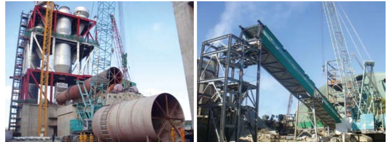
▲ 回转窑吊装 Rotary kiln lifting
