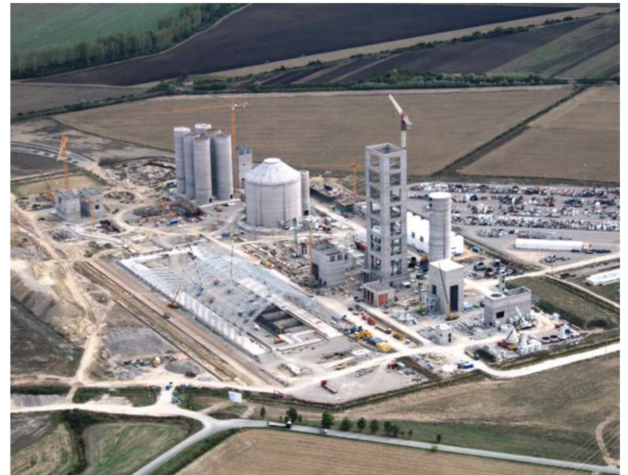
▲ 项目建设过程中的现场 Site during construction
