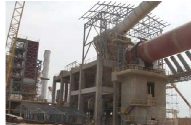
▲ 烧成系统建设 Construction of firing system
