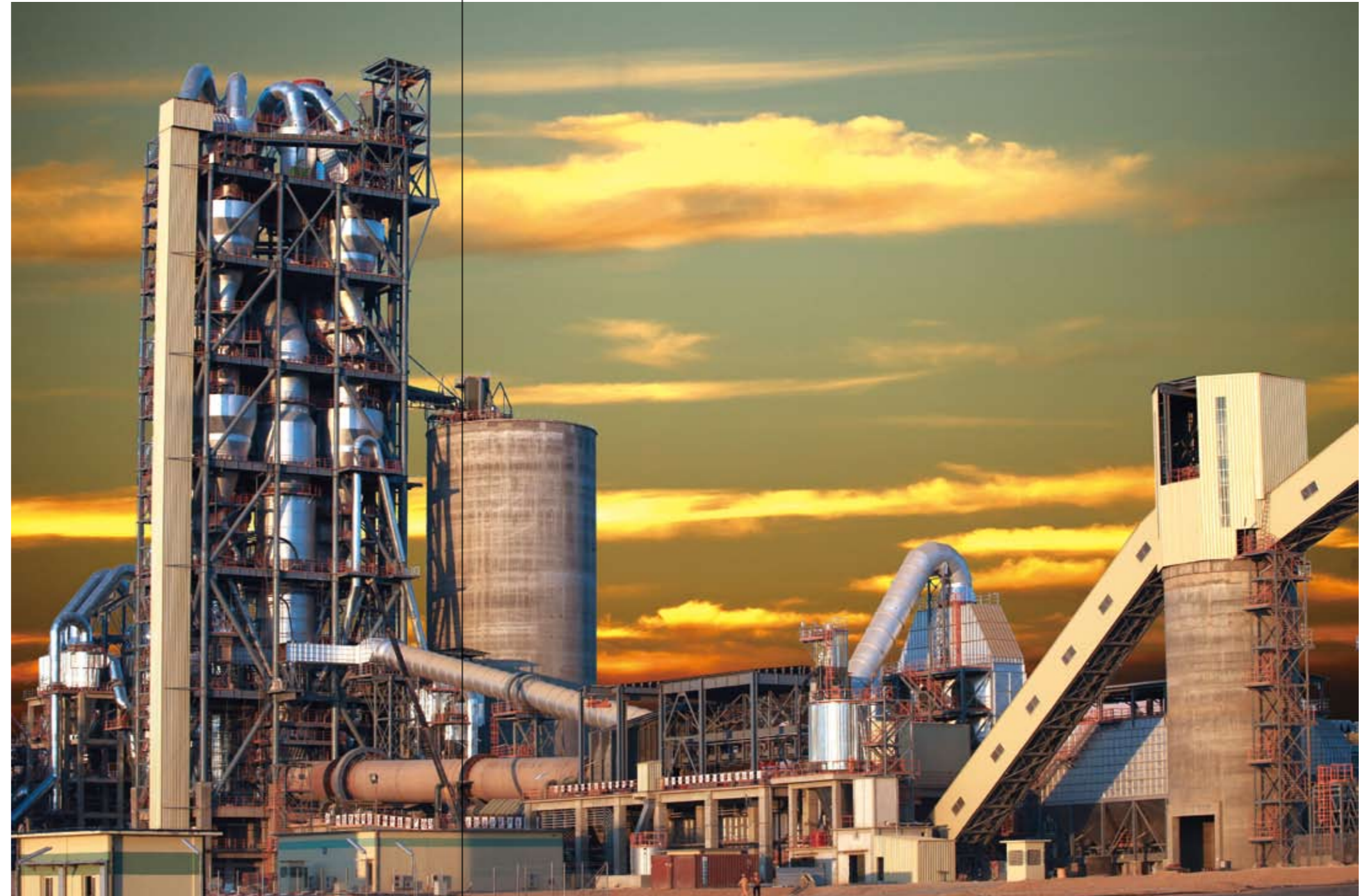
▲ 建成后的叙利亚ABC项目 After the completion of the Syria ABC project
