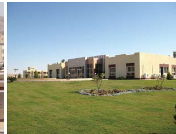
▲ 主行政楼 Main Administrative Building
