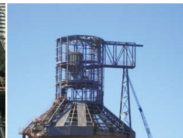
▲ 492熟料库钢构安装 492clinker silo steel installation
