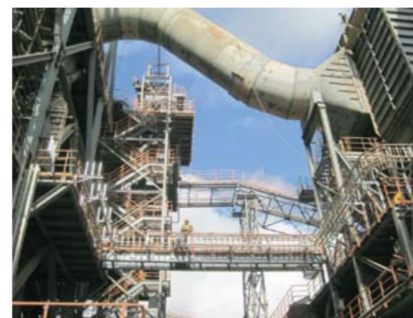
▲ 362原料磨桥架安装 362raw material mill bridge installation
